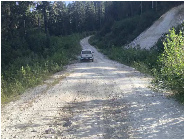
Road over culvert
